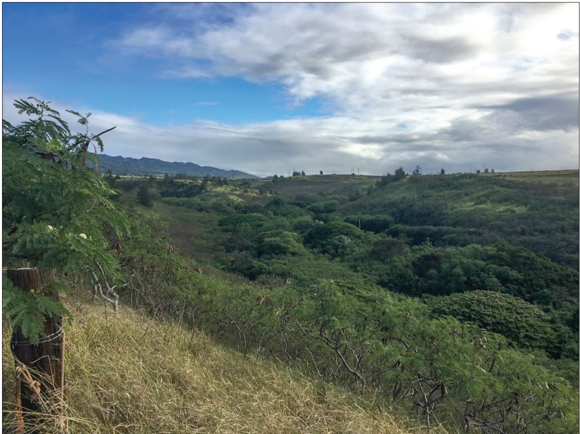
Figure 1. Overview of Honouliuli National Monument, view is northwest towards Compounds I, II, and III, from UH West O‘ahu Access Road; view in foreground is Compounds V and VI. May 2017. Photograph by William R. Belcher.
